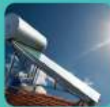
SOLAR WATER HEATER
